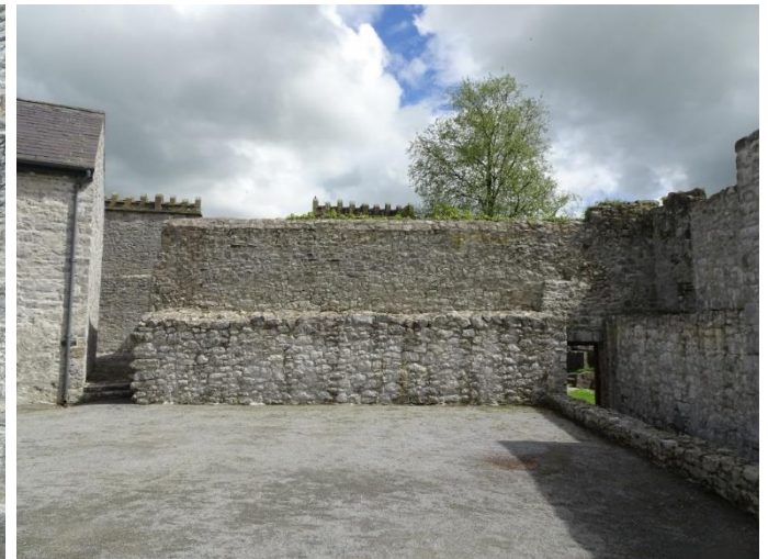
14. Rear of west wall built over medieval castle wall
