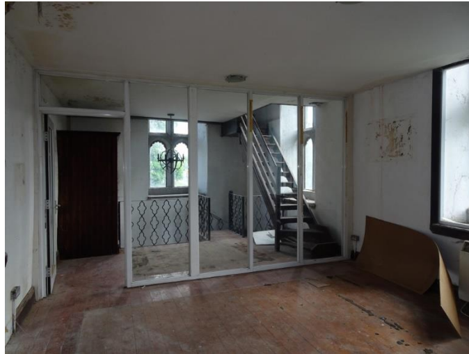
51. First floor looking east
