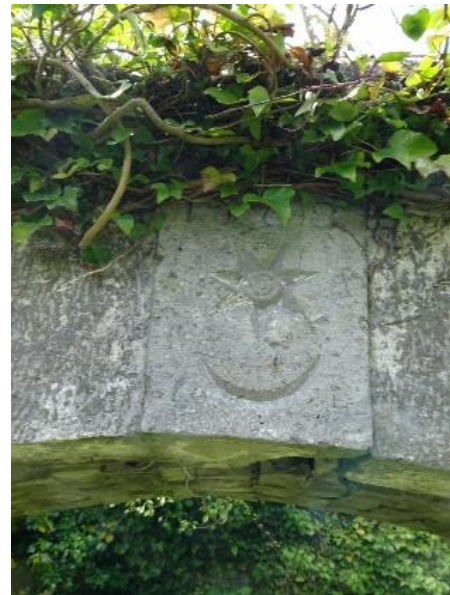
Mason's mark on the keystone of the arch to the rear outhouse
