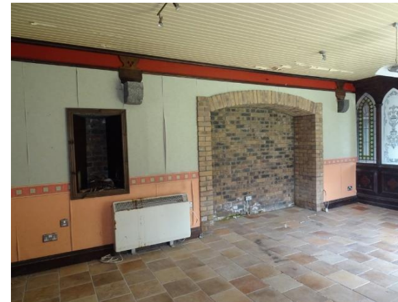
South building ground floor
