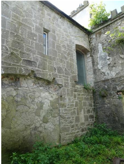
32. South building_north facade
