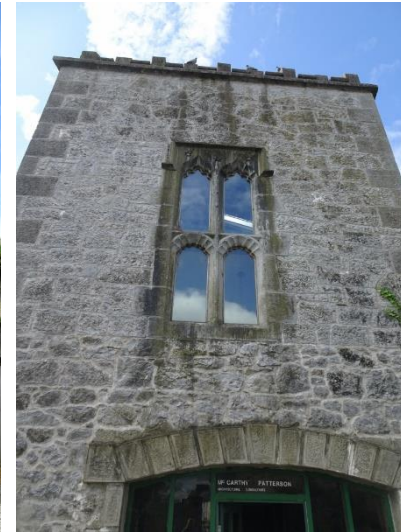
3. Cut stone window at first floor level
