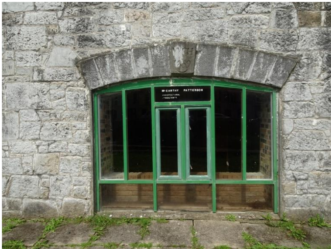
12. Ground floor window_rebuilt arch_date stone WFH 1859
