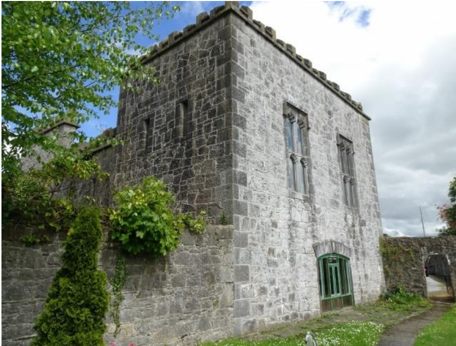
South elevation facing onto the river.
