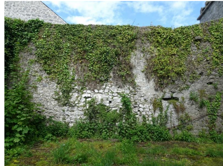
43. North boundary wall
