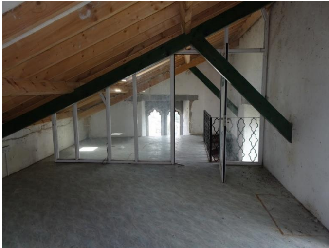
50. First floor looking west
