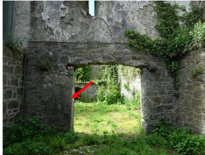
29. West wall of courtyard_note plaster on FF level_arrow locates mason's mark
