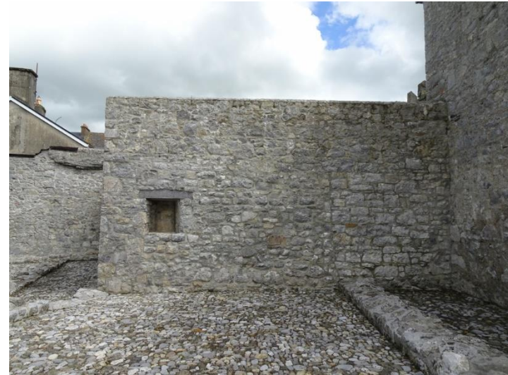
18. L-shaped structure RPS 1489_under separate ownership
