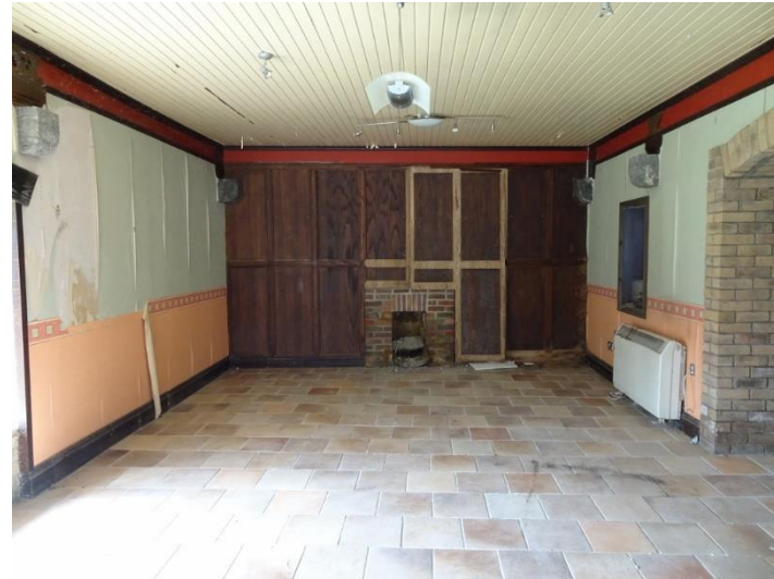
46. Interior of main building_ground floor
