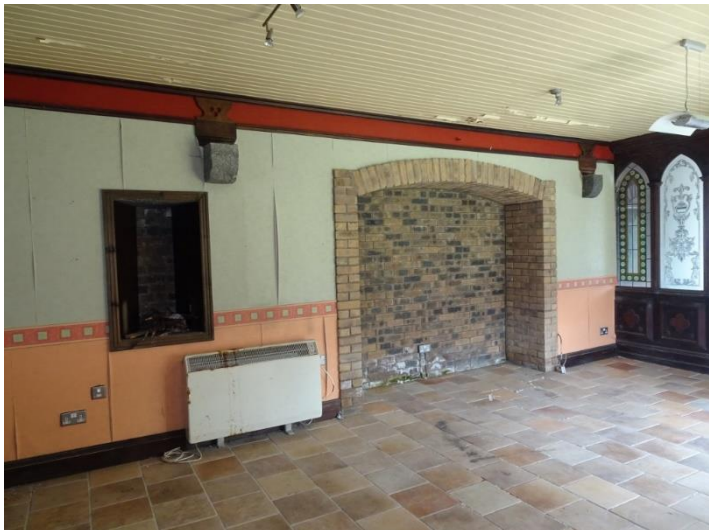
47. Blocked up archway
