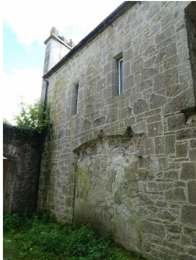
33. South building_north facade
