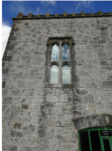
10. Cut stone window at first floor level
