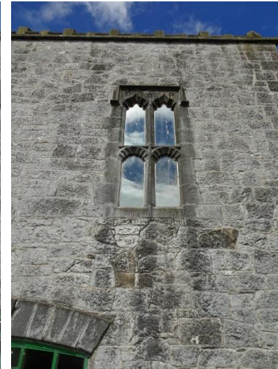
11. Cut stone window at first floor level
