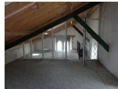
South building first floor
