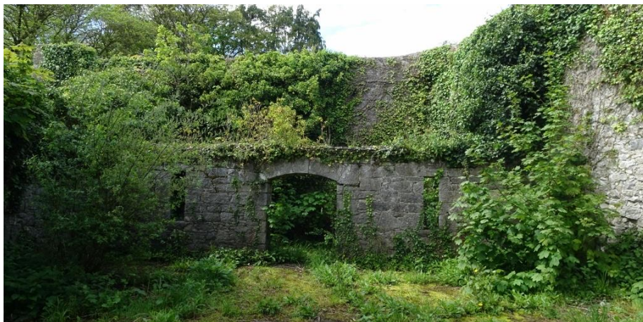
Outbuilding at the end (west) of the garden
