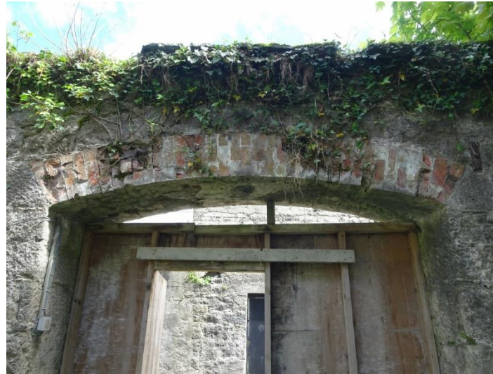
34. Inner face of courtyard entrance arch
