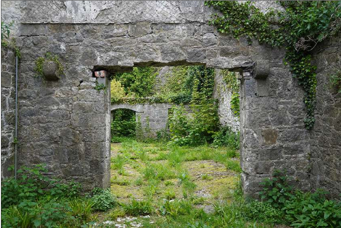
Plate 1. View through arch into courtyard area, from E.
