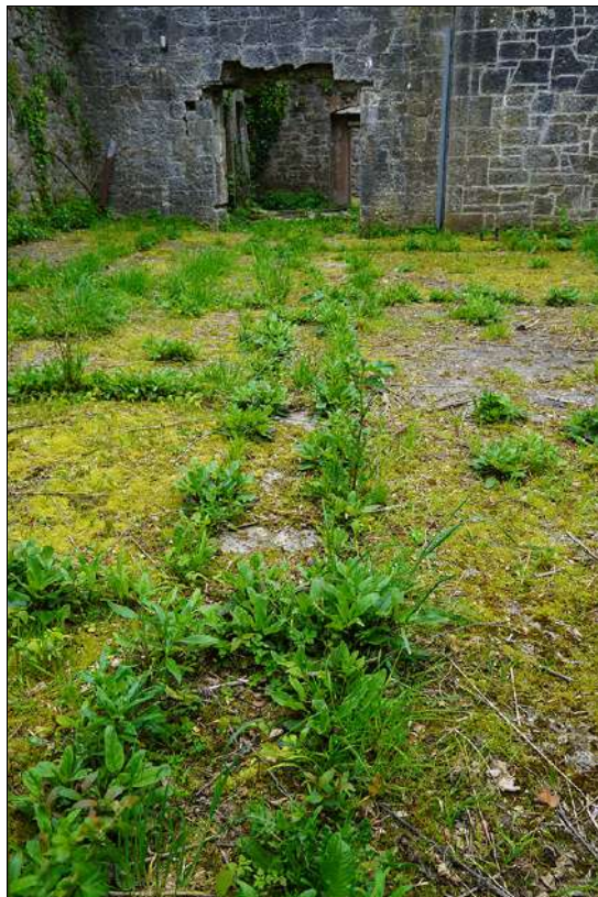
Plate 3. Detail of drains and outline of sheds relating to the use of the site as an abattoir indicated by weeds in cracks in the concrete, from E.
