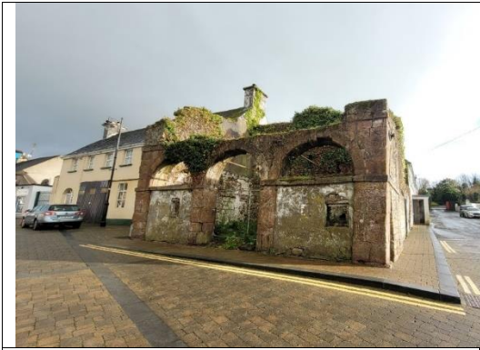
Image 1-1: View of derelict building from the front
