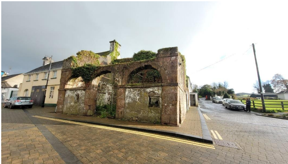
Image 4-1: View of derelict building from the front
