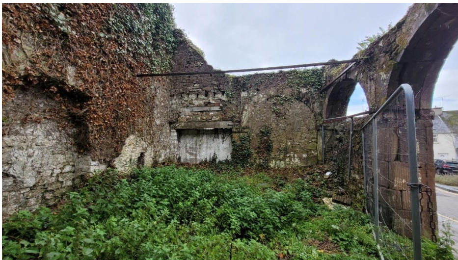
Image 4-2: Internal view of the building space
