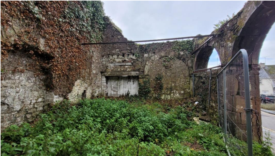
Image 3-2: Internal view of the building space
