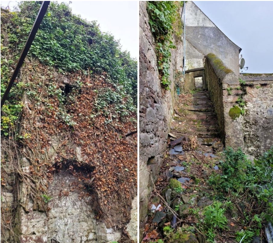
Image 3-3: Ivy covered internal wall and stone steps to the rear of the building.
