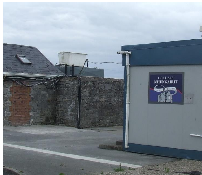
D9: Wall (C)fig.03- South Inner wall ( C) / South Elevation Building K
