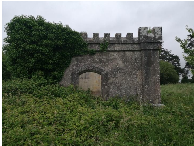
C7: West Facing Elevation, indicating main entrance door.
