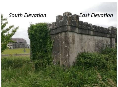
Fig.11d Survey photo: Observatory South & East Facing Elevations
