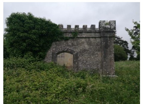
Fig.11e Survey photo: Observatory West facing Elevation
