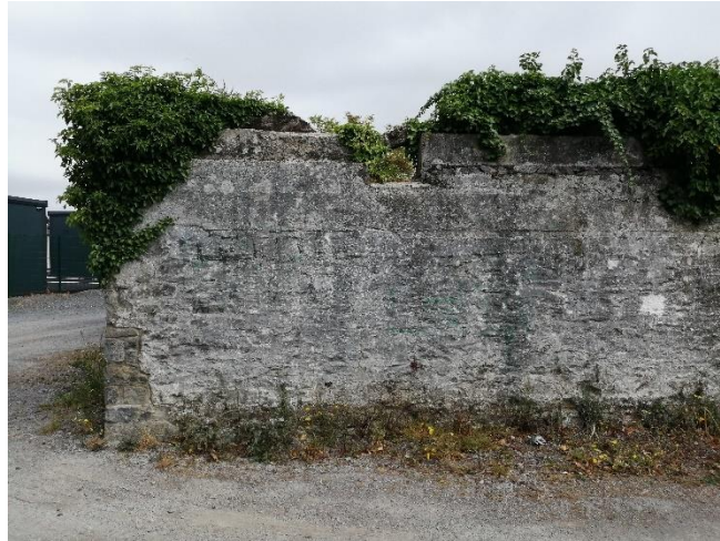
D4: South/West Boundary Wall
