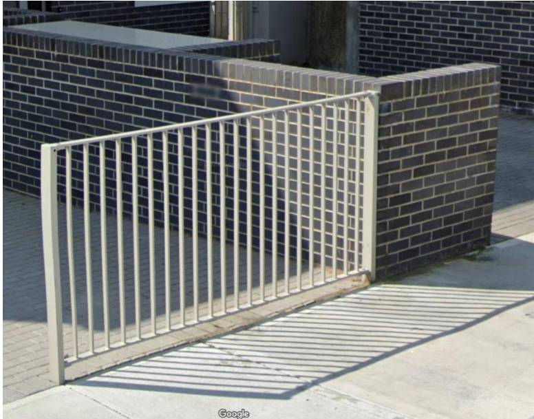
Figure 7.0 – Boundary railings style.
