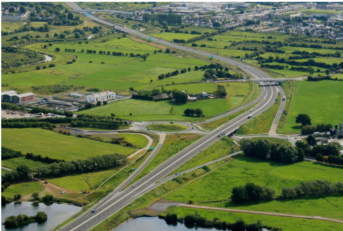
View of the Limerick Southern Ring Road Phase 2, Bunlickey Lake in the foreground, Ballykeeffe in the Background
