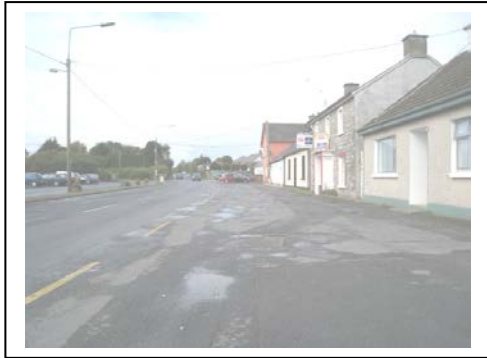
Figure 10.24 Village centre prior to 2013 improvements
