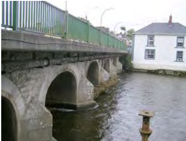
Figure 17: Croom Bridge, Protected Structure Reference 1133
